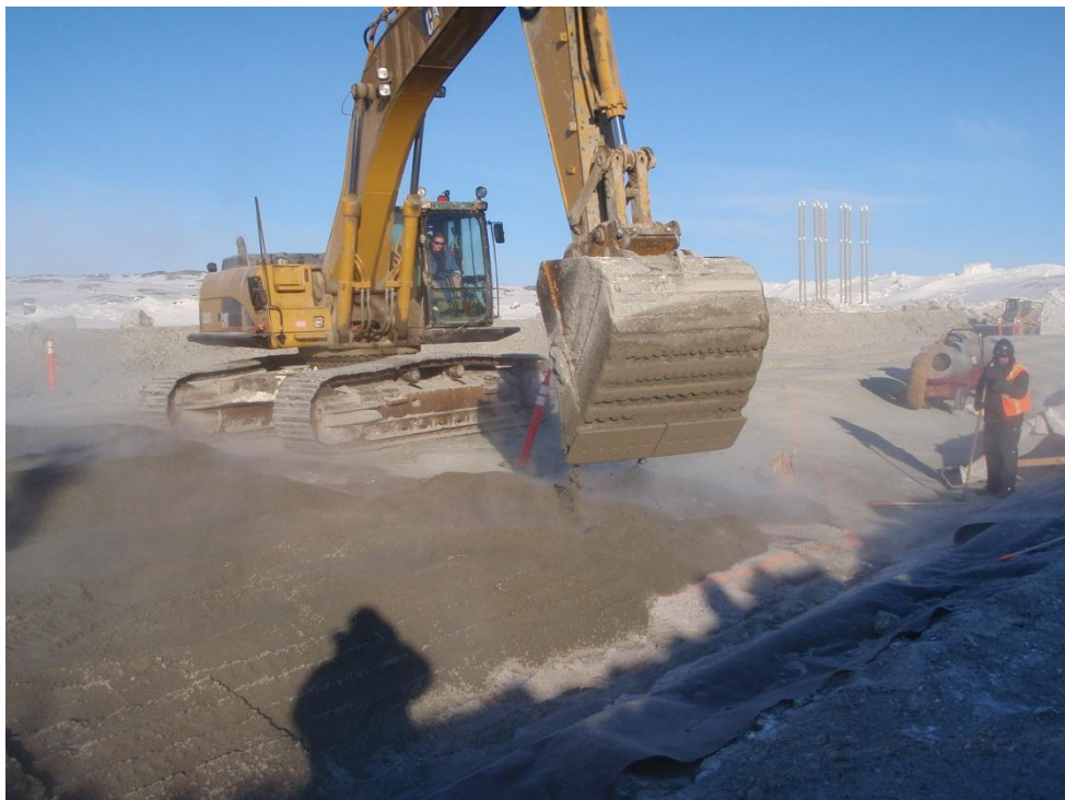
Photo 5: Covering thermistor cable at chainage 1+30
